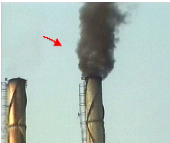
Soot Blowing Before EGS HEAVY
