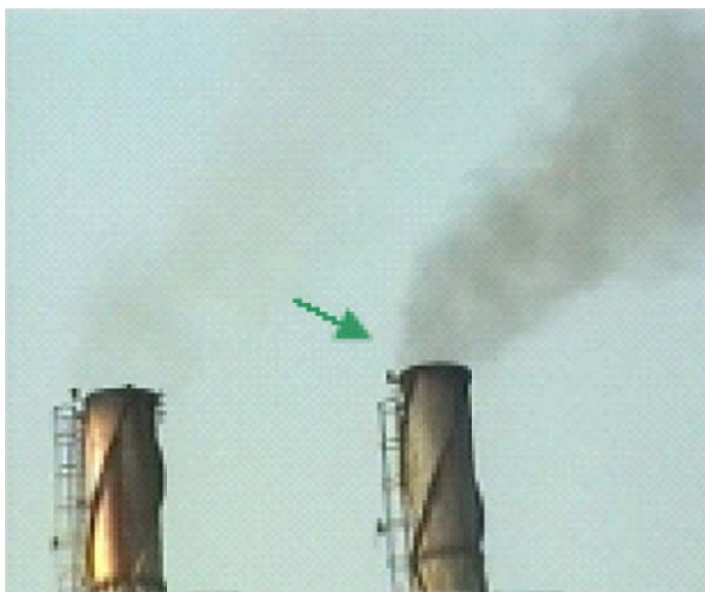
Soot Blowing After EGS HEAVY
